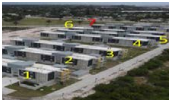
Nelson Mandela University – bird's eye view of student accommodation (blocks 1 to 6 completed for occupation in February 2023)
