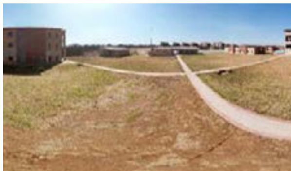
North West University – panorama view of completed student accommodation blocks
